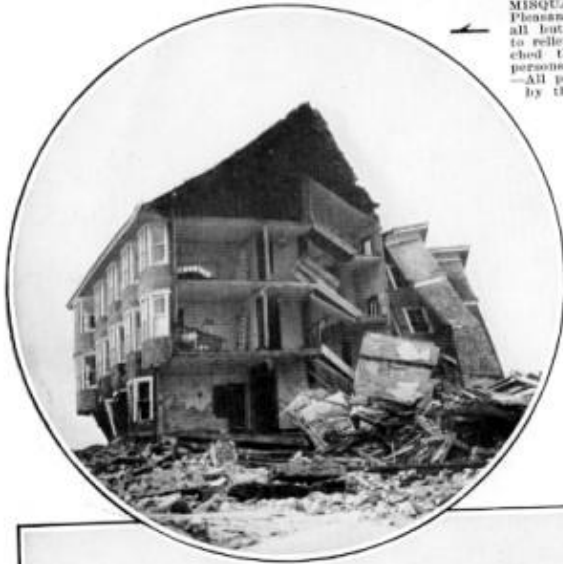
POINT O WOODS, CONN. This row of cottages, all of which were built within the year, were almost completely destroyed. Note the ones pushed back from their concrete steps.
