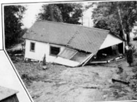
HIGGANUM, CONN. This building was undermined by flood waters before the hurricane and then blown away by the great force of the wind.
