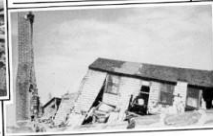
HIGGANUM, CONN. This building was undermined by flood waters before the hurricane and then blown away by the great force of the wind.
